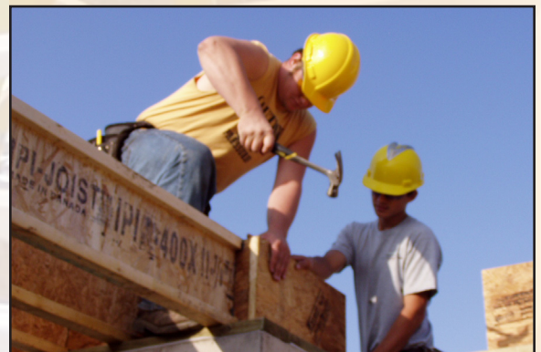
Hands-on learning experience makes a difference to employers seeking to employ framers and other construction workers.
